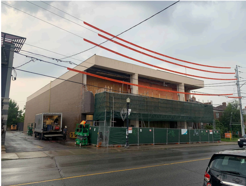
Hoarding on the front of building
