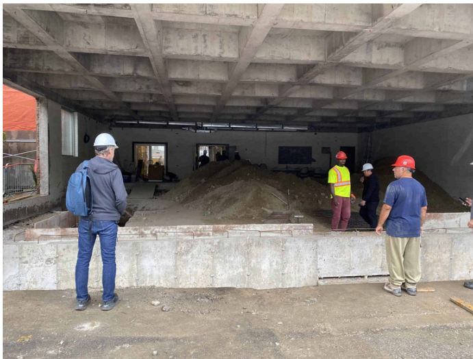
The west meeting hall on the ground floor under the old loading dock
